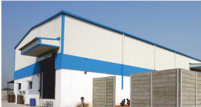
Production Plant at Rohisa, Mehmedabad, Gujarat
